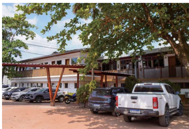
Administrative Facade in Belém, Brazil. Photo: Fernanda Tocantins
